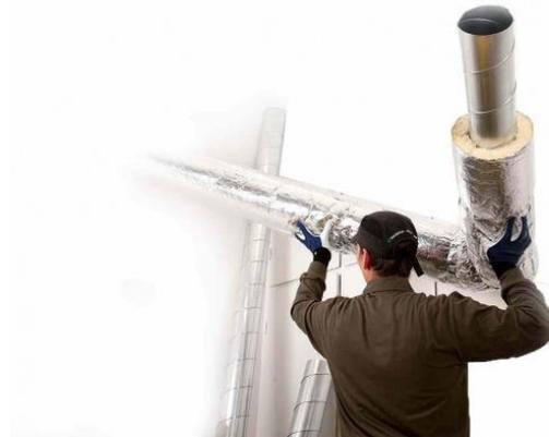
In areas with extremely low winter temperatures, additional insulation must be used. Total insulation thickness must be at least 100 mm.
